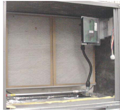
Fig. 77 - Return Air Sensor Operating Position
