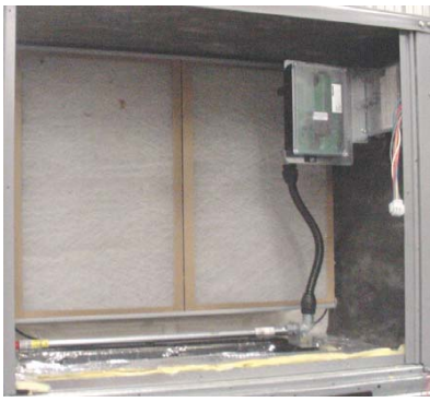
Fig. 23 – Return Air Sensor Operating Position
